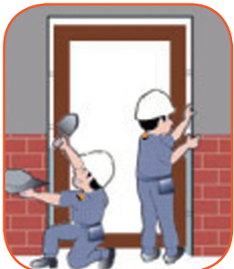
3. Filling around the door frame
